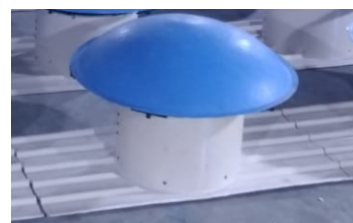
Motorized Roof Exhaust Fans
