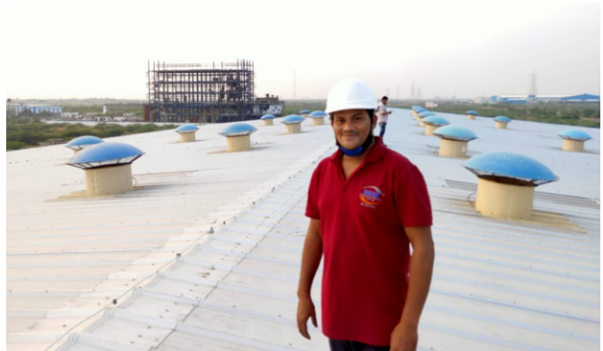
MOTORISED / FRP BASE ROOF EXHAUST FANS
